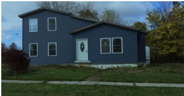
Figure 2.4. One Resident’s Self-Built Home. For over a decade, a longtime Heights resident built this house from right to left and by their self. When the 2007-2009 recession hit, the resident and their family lost the house; soon after, a white couple moved in. Source: Picture from “Small Community Redevelopment Toolkit” (2014)
